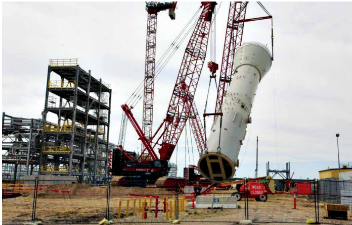
Early in July a pair of large-scale cranes working in perfect unison hoisted our new 280-tonne, 38-metre-high polyethylene reactor into place.
